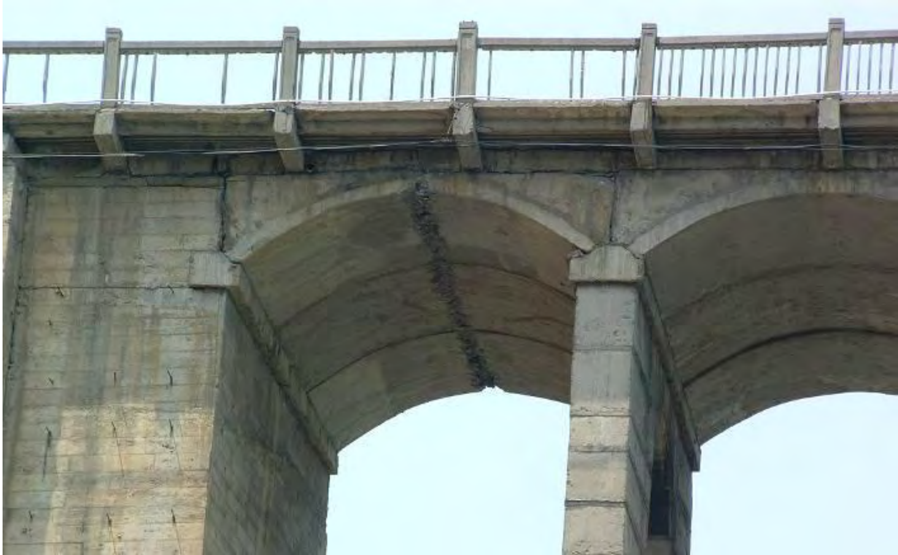
Crushing of concrete in spandrels
