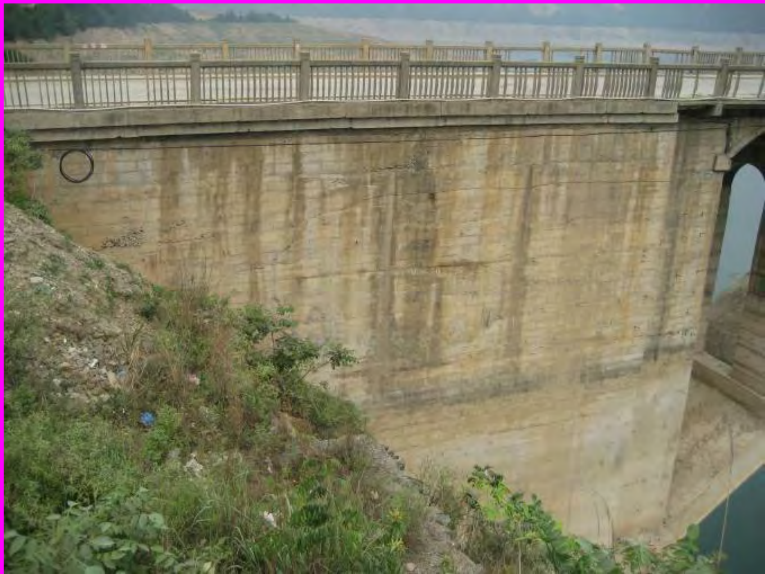
Crack in abutment
