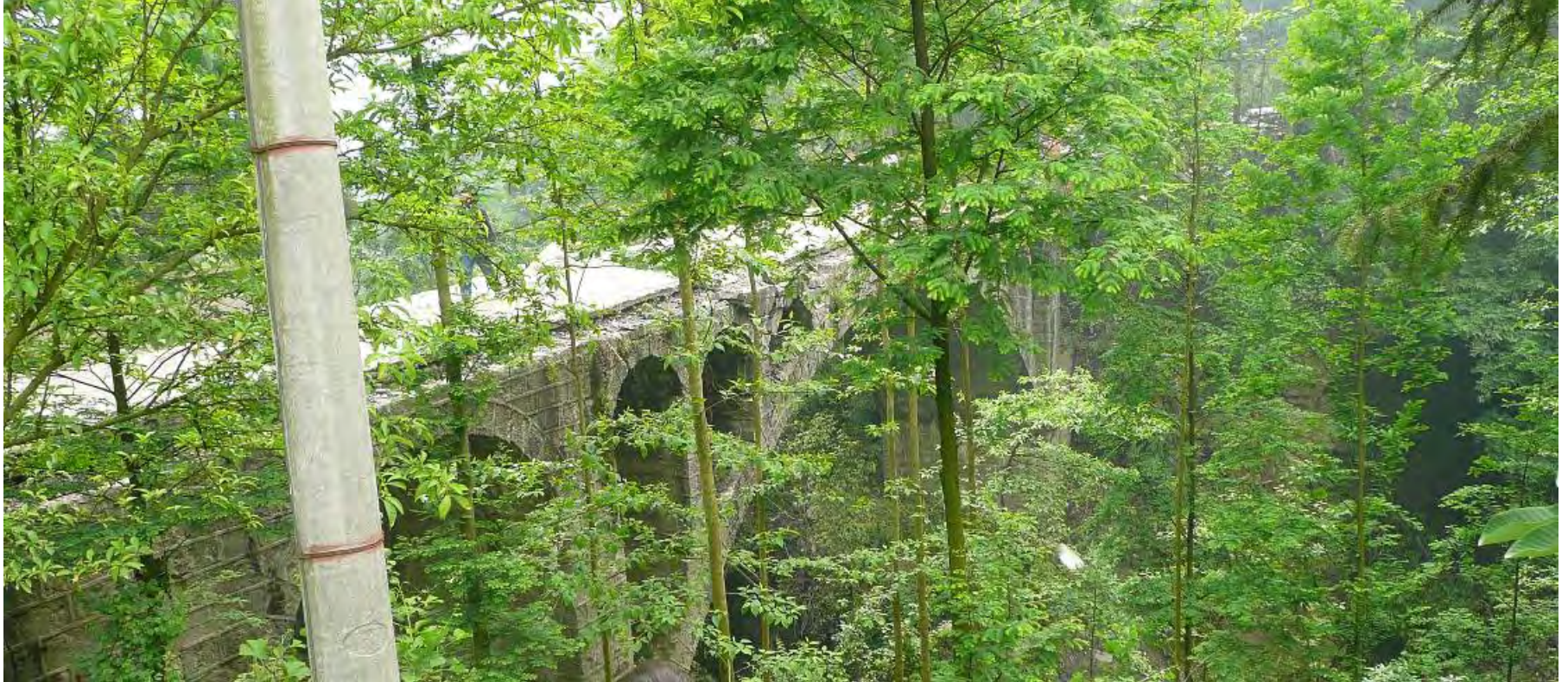
Masonry arch bridge
