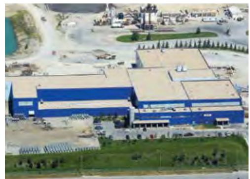
Spyhill plant, Calgary, Alberta
