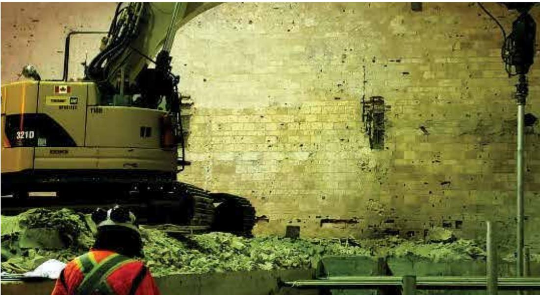
*VersaPile, Inc. installed 64 helical piles to till for Concord Projects inside of the iconic Academy Lanes building in Winnipeg, MB to support its conversion to multi-family condominiums. Air scrubbers were added to the equipment and the supervising engineers were able to monitor the installation torque on their phones using a Wifi connection to VersaPile's Intellitork torque monitoring system.*
